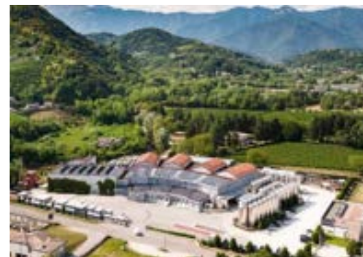
Facilities Collection center, vinification, sparkling and bottling plant in Pieve di Soligo
